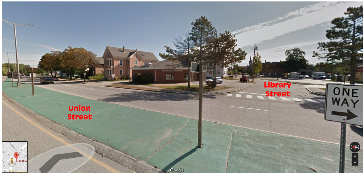
View from Union Street median looking down Library Street.
